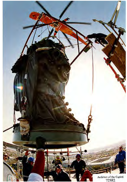
A sky crane helicopter replaces the conserved bronze Statue of Freedom atop the U.S. Capitol. This photograph was taken by a remote camera. PTIB uses remotely triggered cameras for many tasks. AOC Photography, 10.23.1993
