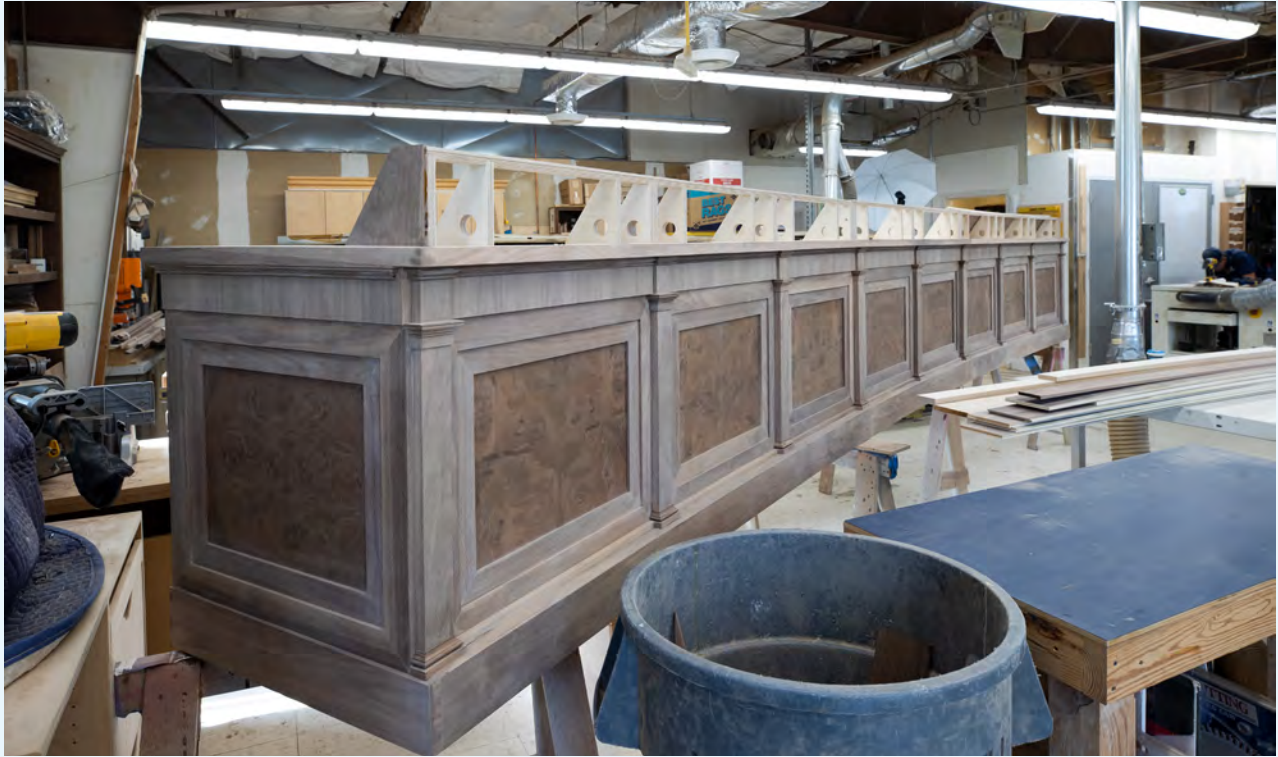
A section of the new dais is constructed in an AOC wood shop. This model will serve as a prototype for future renovations.
